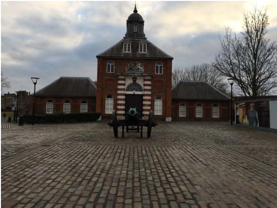
The main entrance of the old Arsenal of Woolwich
